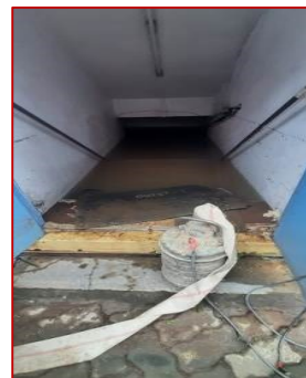
Water being pumped out of the basement
